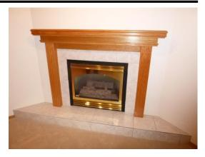
Type: Gas log direct venting with pilot light.
